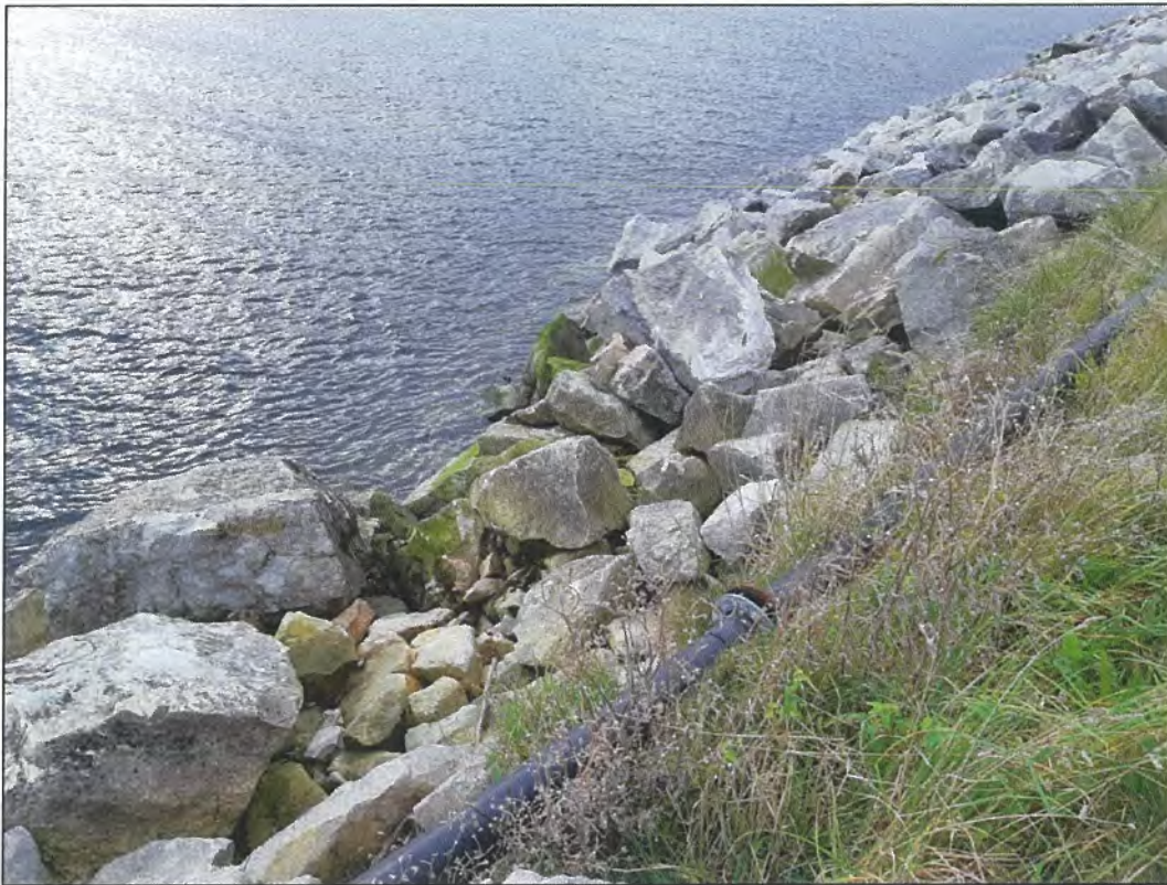
Floodwall batter before repair.
