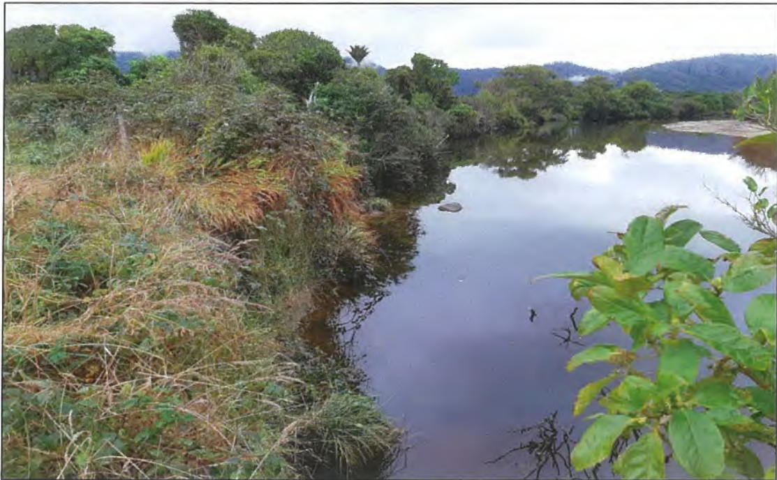
Bank slumping on the Oparara River.
