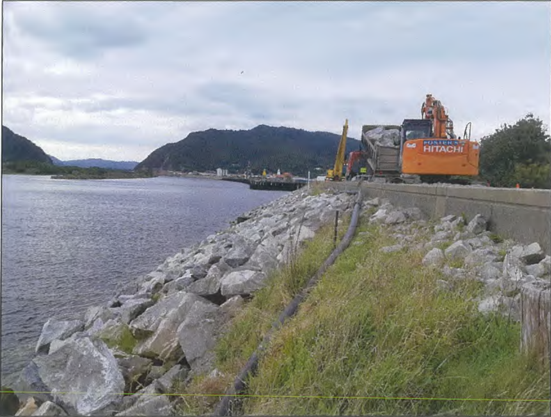
Extension of the rock riprap at Blaketown.
