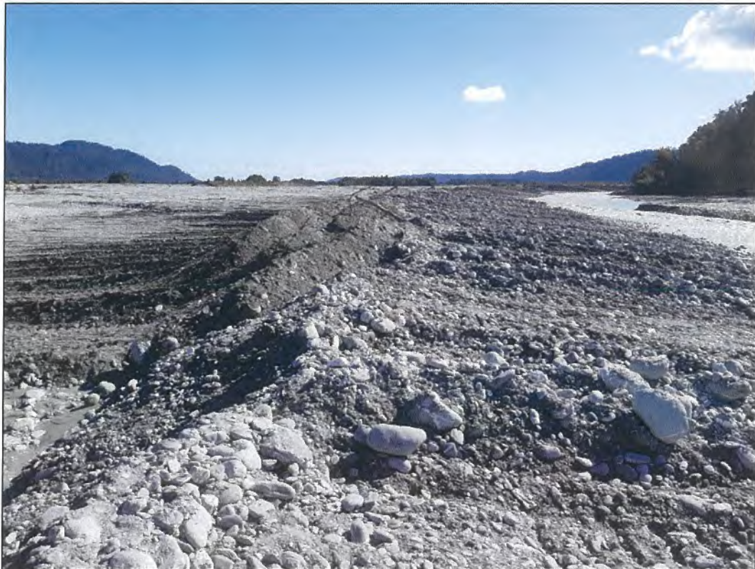
Temporary river diversion Lower Waiho.
